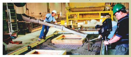
WINDOWS AND DOORS ARE PLACED on the casting bed before the concrete is poured.
