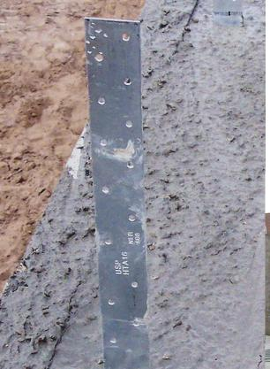
HURRICANE STRAPS, like those shown at left, are wet-set into concrete walls at strategic locations. In addition, the building envelope was improved through tight concrete construction, shown below left, and continuous foam insulation boards adhered directly to concrete walls as shown below.
