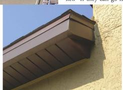
**EXTENDED FASCIA DESIGN**, above, creates a drip edge to drain water out and away. Baffled roof vents, above right, make it more difficult for rain to penetrate into attic spaces.
